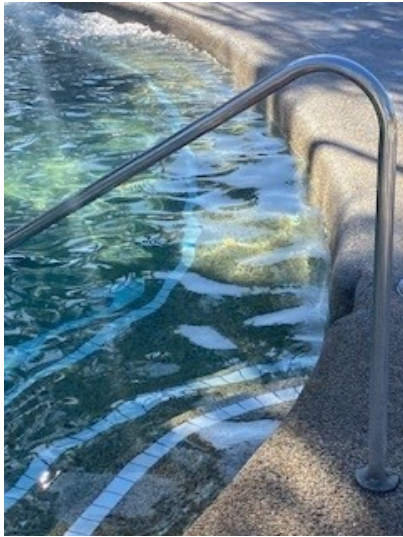
Handrail into pool
